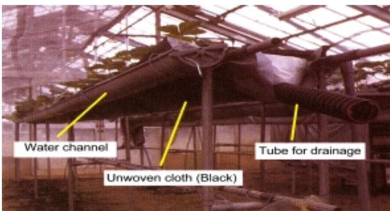
Fig. 2. Evaporative cooling system
