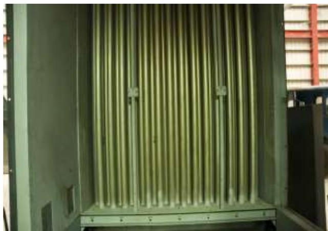
Fig. 10. The heat exchanger. (Suncue, 2014)
